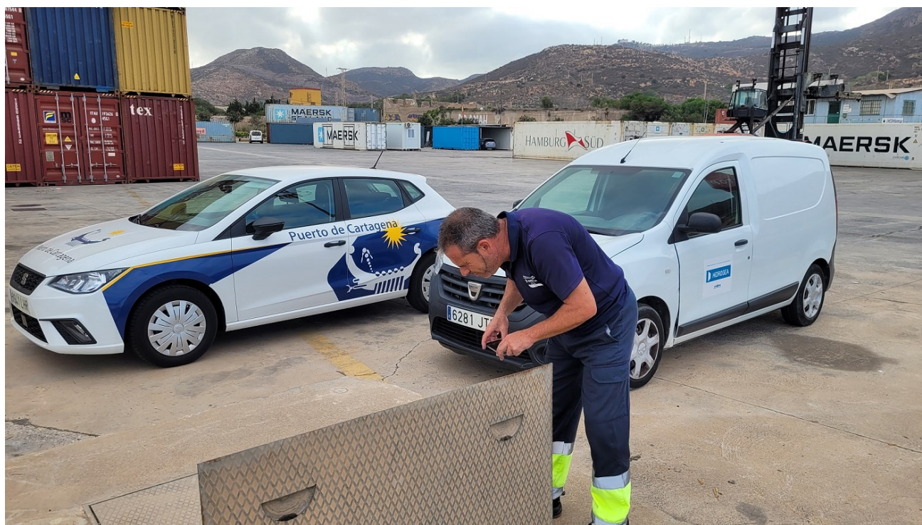
ECA inspection of the two pumping wells in the Cartagena basin, carried out by MUNUERA Laboratories and verified by Hidrogea
