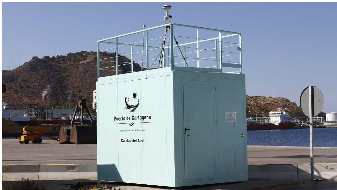
Metering station at Principe Felipe-Isaac Peral docks
