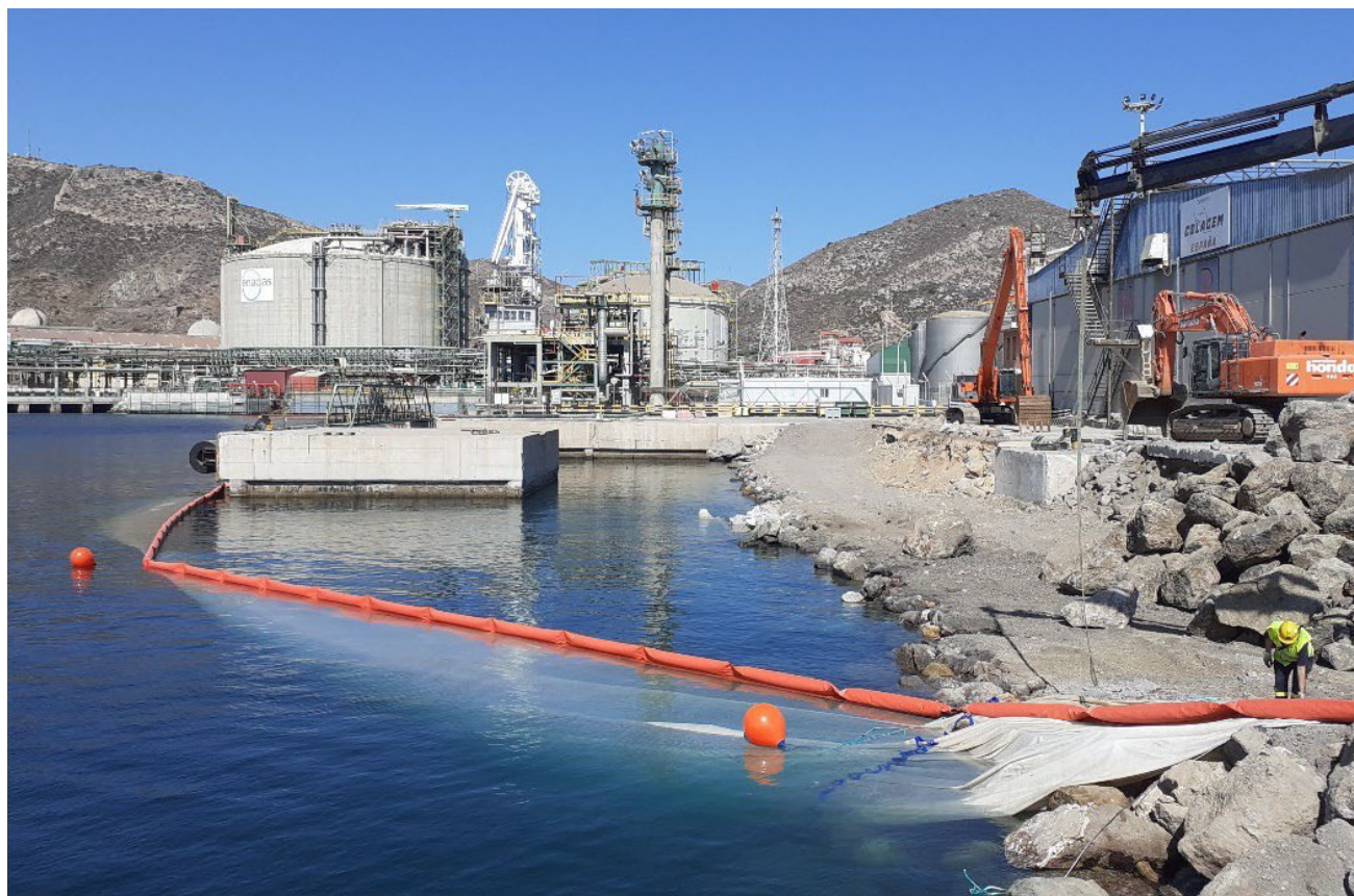
Anti-turbidity barrier during the LNG loading dock expansion works in Escombreras
