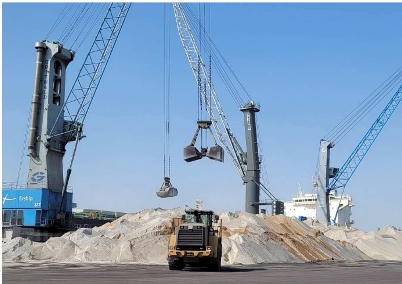
Loading of aggregates in Escombreras
