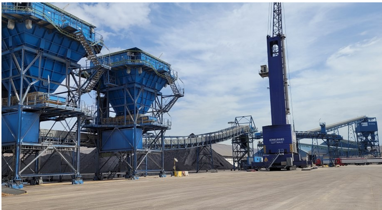
New conveyor belts and eco-friendly hoppers to minimize particle emissions installed by Ership, S.A.
